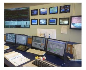
SCADA systems are typically supplemented with a process historian, which is used to archive sensor values, setpoints, and alarms for later analysis and real-time trending. For A&S Energie, their systems produce about 2,000 relevant data points at 1 second resolution kept in long-term storage.
